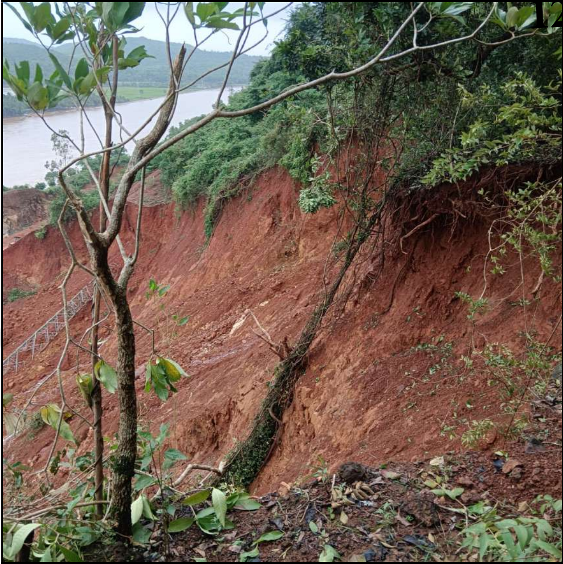
Fig. 1.13: Thickness of overburden at the main scarp
