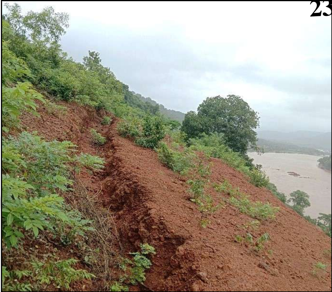
Fig. 1.15: Trenches observed above the Ch. no. 147.500
