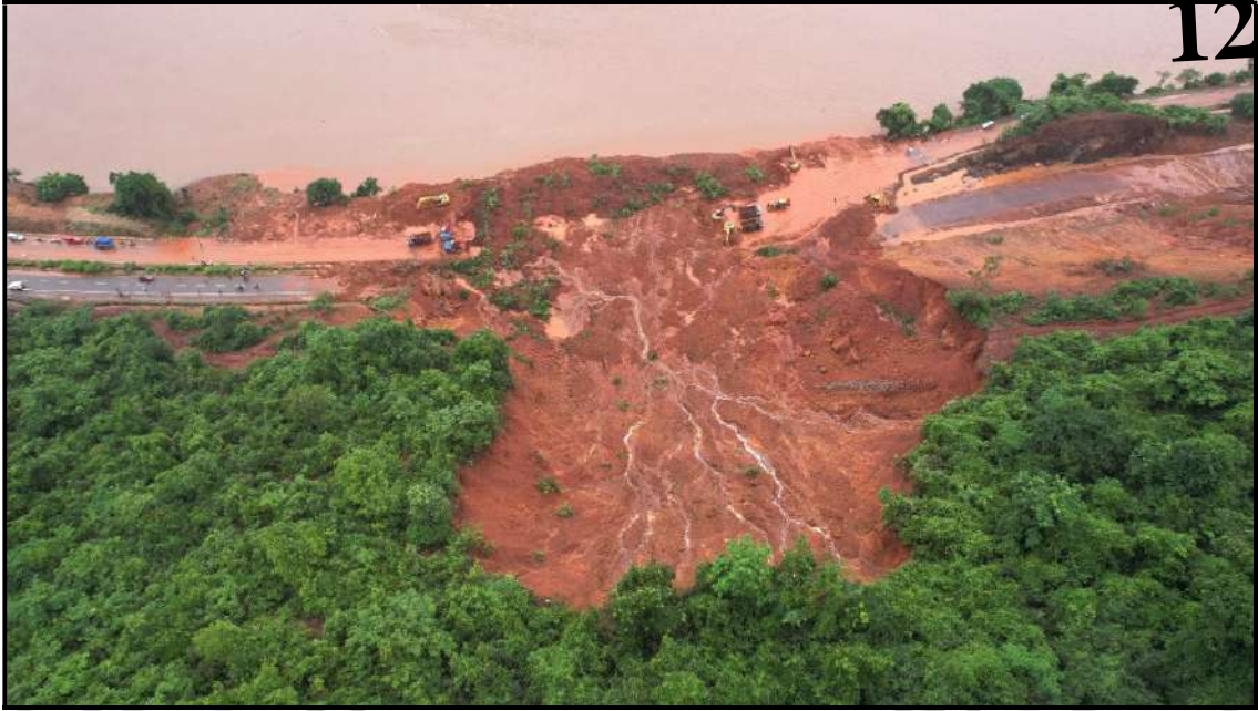
Fig. 1.2: Aerial view of Shirur landslide blocking the communication corridor NH-66 (courtesy IRB)
