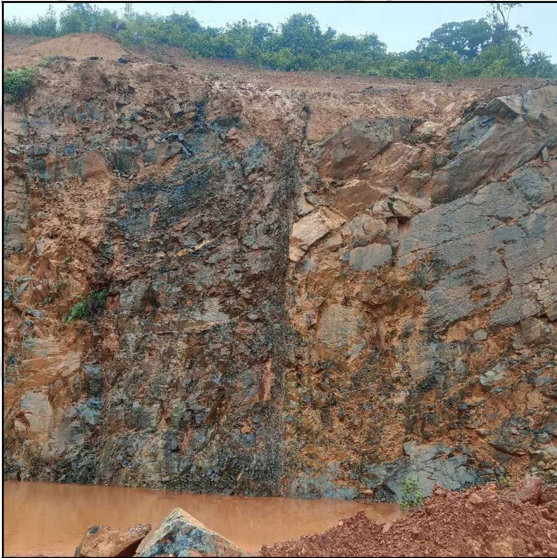
Fig. 1.5: Minor Fault observed at the base of the cut slope on the right flank of the slide
