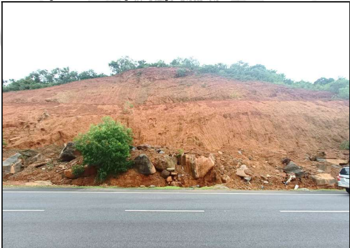
Fig. 2.8: Slope cut at chainage 168.200 exposing lithomarge and debris
