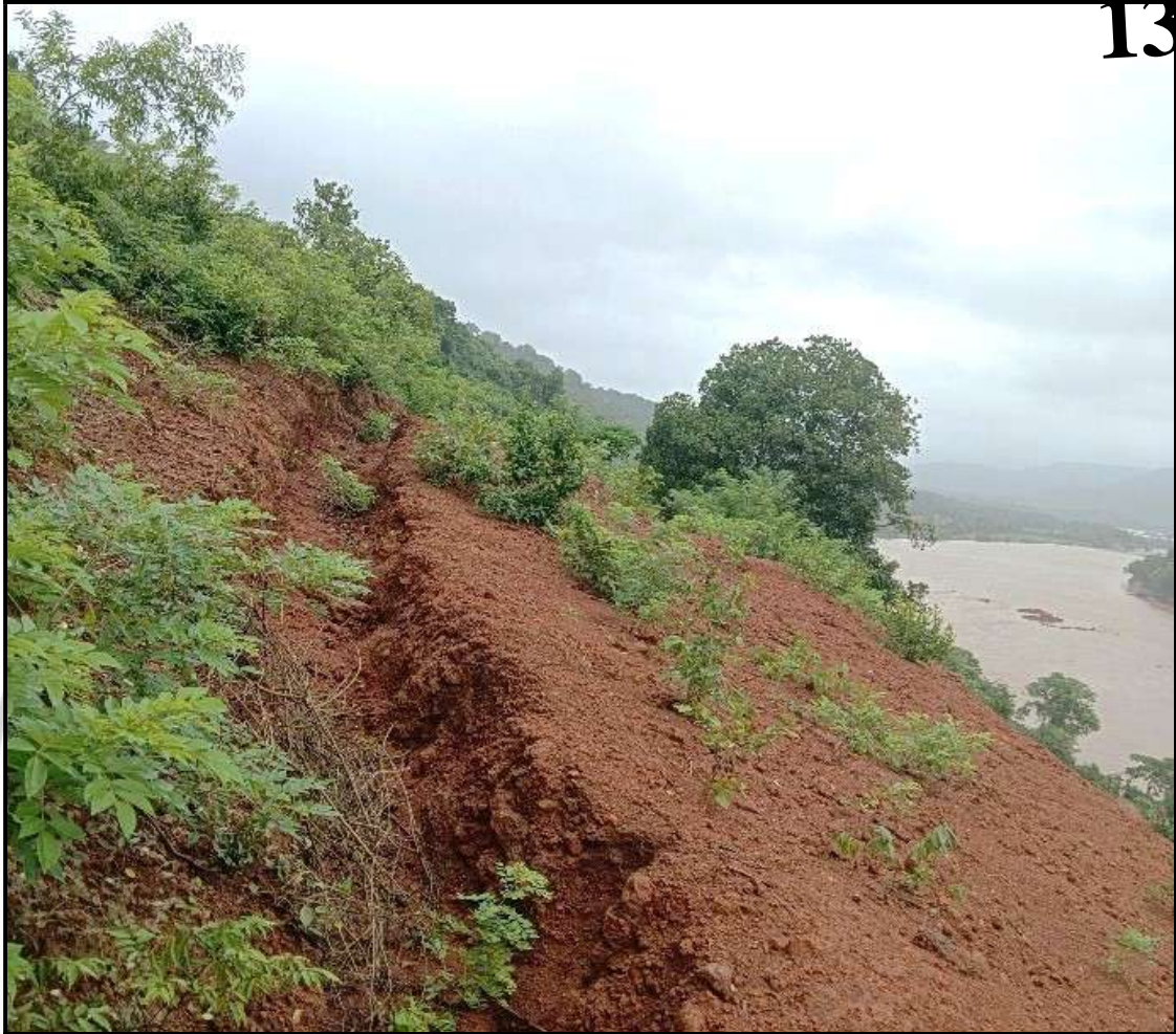
Fig. 1.15: Trenches observed above the Ch. no. 147.500
