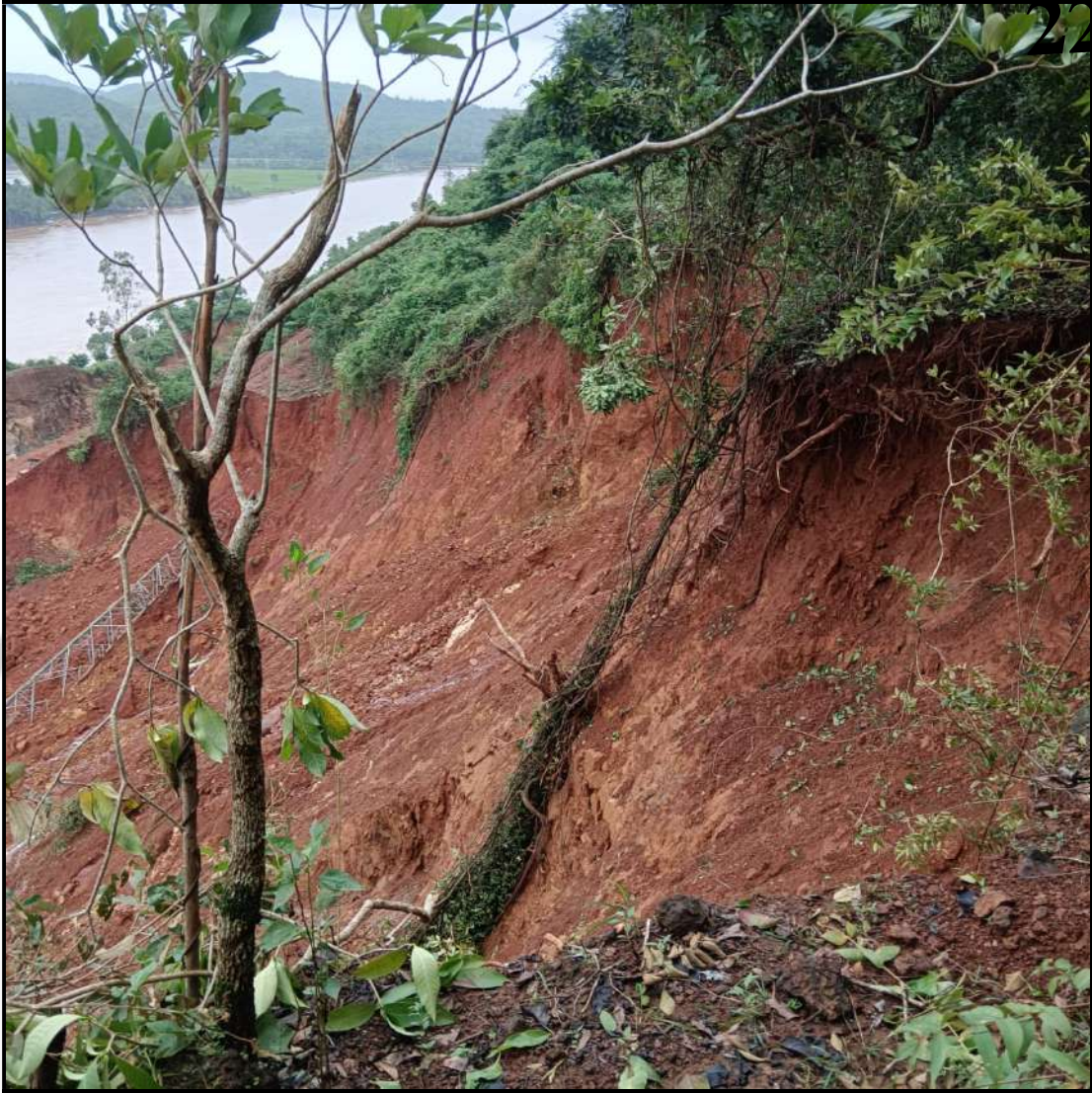
Fig. 1.13: Thickness of overburden at the main scarp
